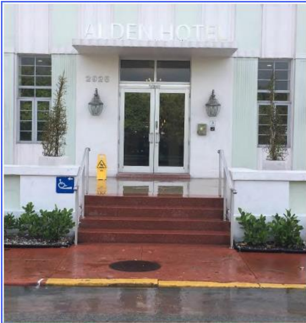
Figure #16. Photograph taken the morning of October 16, 2016 by Coastal Risk Consulting, Inc. documenting conditions in front of the Alden Hotel at 2925 Indian Creek Drive during a King Tide event.
